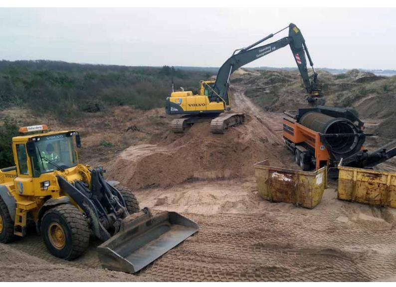
Removing Japanese rose at Haversdal nature reserve in Halland using a wheel loader, excavator and sorting machine. Here, the deepest roots were several metres deep in the sand since the bushes established themselves in tandem with being covered by drifting sand.
